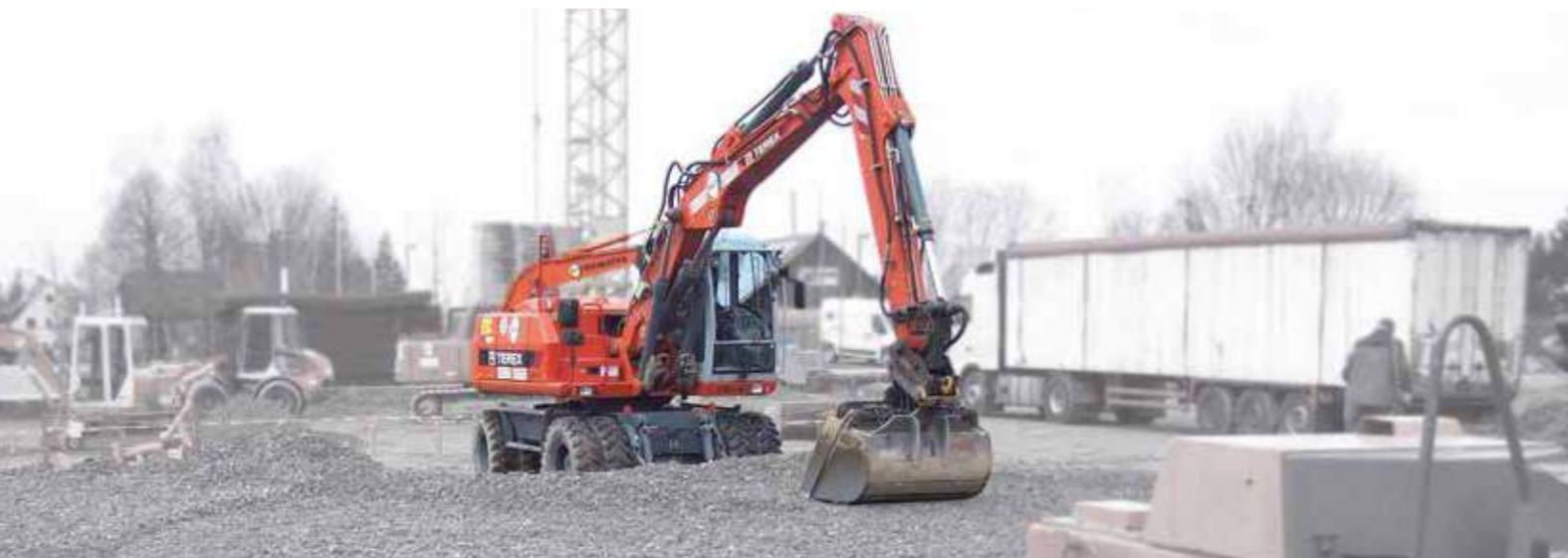
Extensive installation of GEOMATERIALS foam glass gravel for a production hall
