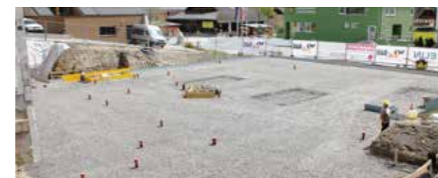
Picture: Primary School in Unternberg, Salzburg © WISA-Bau GmbH, GEOMATERIALS
