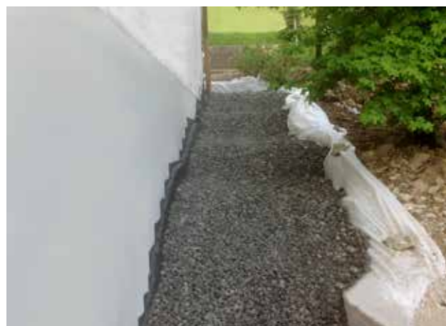
Filling in the working pit and compressing GEOMATERIALS foam glass gravel in layers
